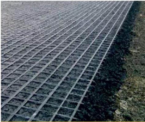
GEOGRID - ASPHALT CONCRETE
