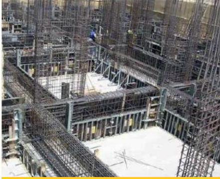
FOOTING AND WALLS
