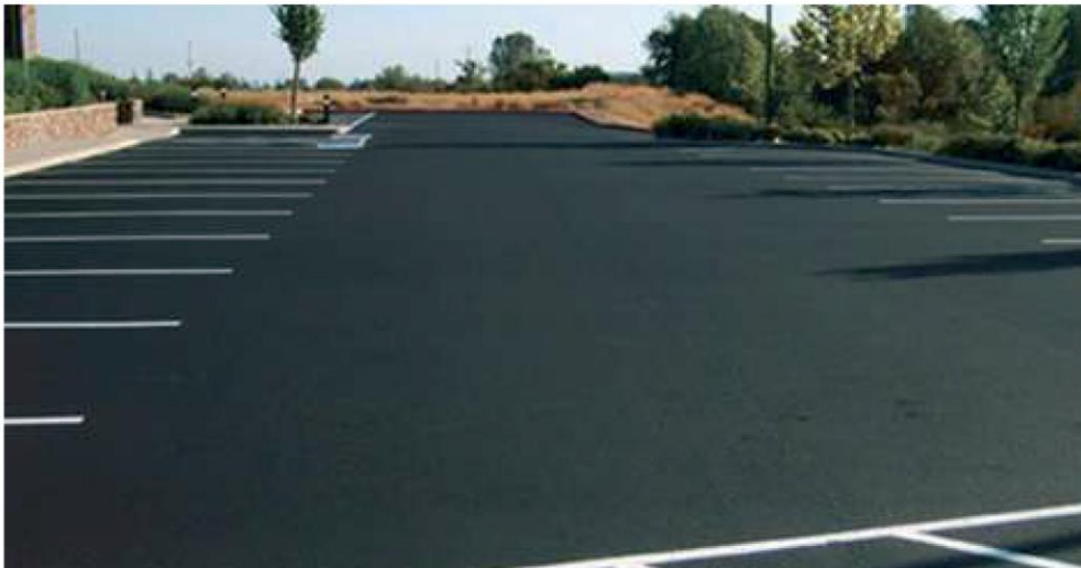
ASPHALT CONCRETE PAVEMENT
