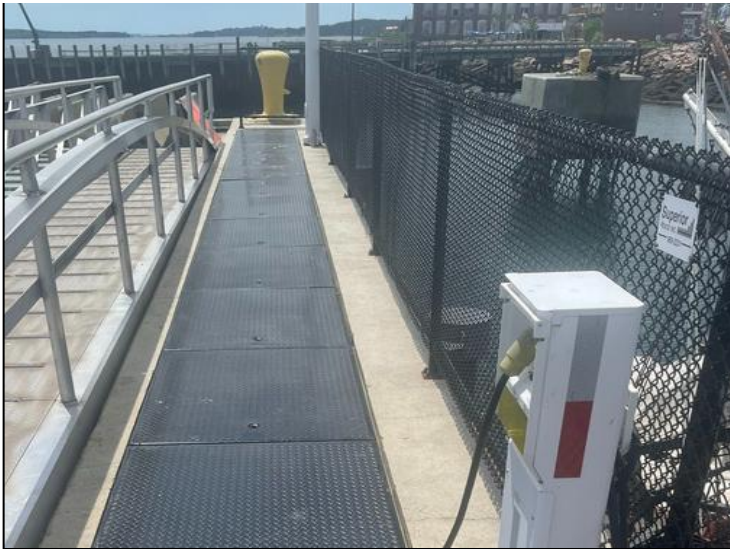
TRENCH COVERS ON THE PIER EASTPORT, ME
